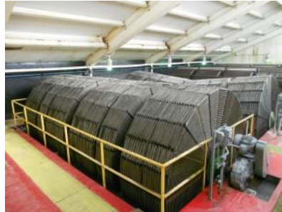
Figure 22 (Courtesy of Skaneateles Wastewater Treatment Plant)
